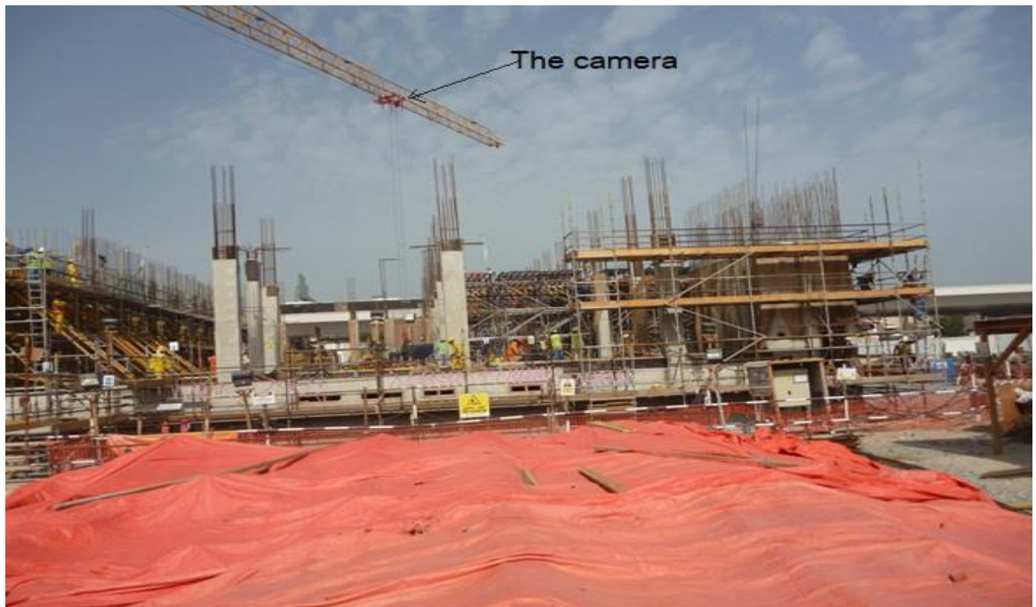
Figure 7. 8: Camera installed on the tower crane
