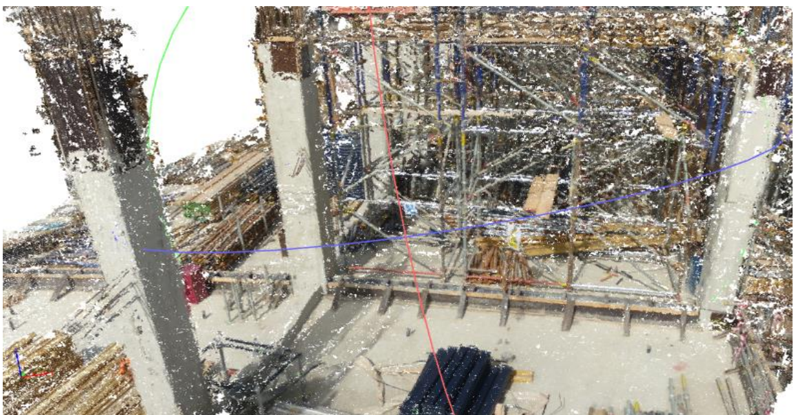
Figure 7.17: Sample of captured site photos with dynamic occlusions used to construct point cloud model
