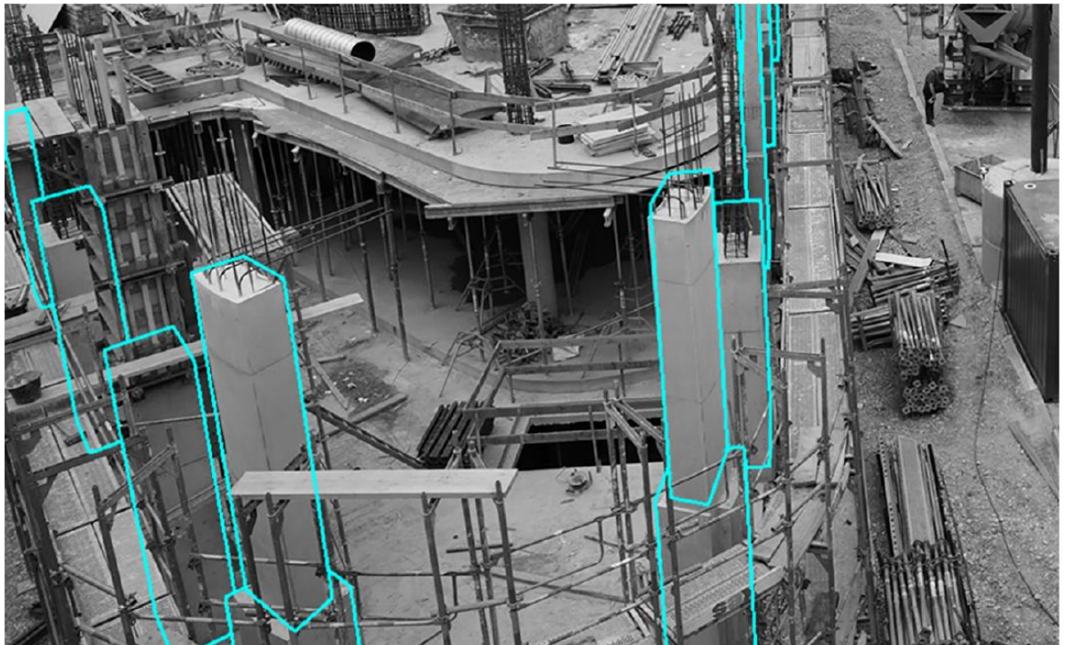
Figure 3.18: Projection of BIM elements onto the captured photo
