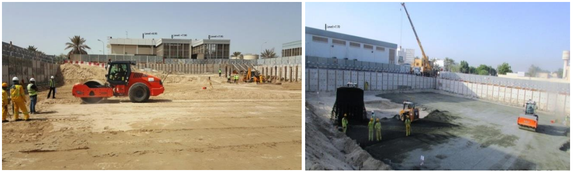
Figure 8.6: Existing buildings close to the construction site
