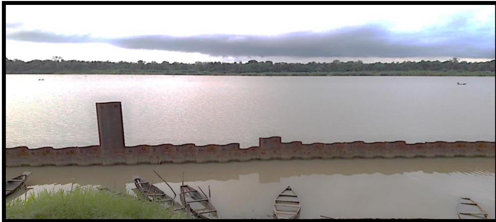
Figure 5.19 Example of Piling Sheet used at the riverbank and canoes used for moving during the flood season at Tombia Community.
