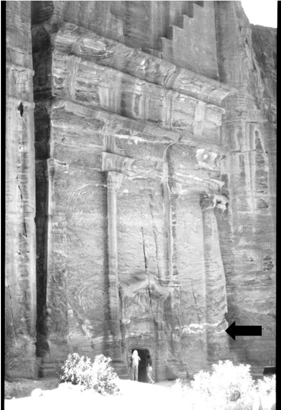
Figure 5: Weathering damage on the facade of the temples of Petra; the arrow indicates the capillary rise to above human height, illustrating the possibility of deterioration from soluble salts.
