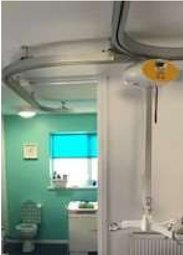
Image 1 Ceiling tracks and hoist (no sling). Note the hole cut out of the top of the door for these to pass through.
