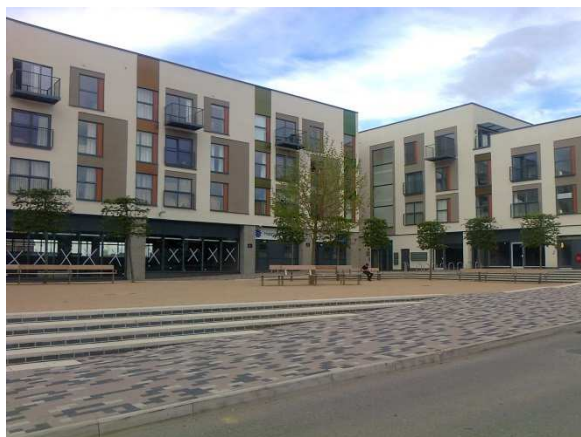
District Centre (not yet fully occupied)
