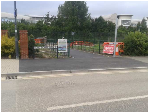
Footbridge looking towards the MoD
