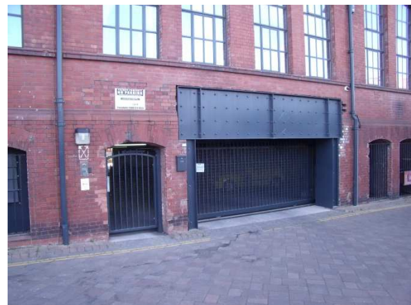
Access to internal car parking
