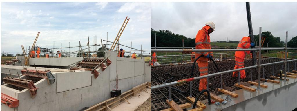
Figure 6. Bridge under construction during deck casting
