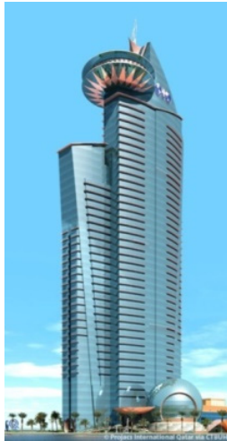
Figure 1: A view of the case study tower (taken from http://www.skyscrapercenter.com/doha/world-trade-center-doha/9918/ ).
