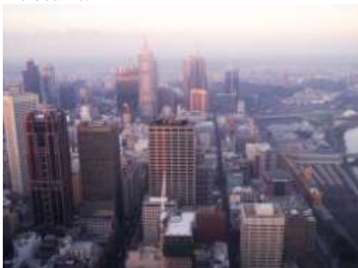
Figure 2: Melbourne CBD showing typical rooftops with Yarra
