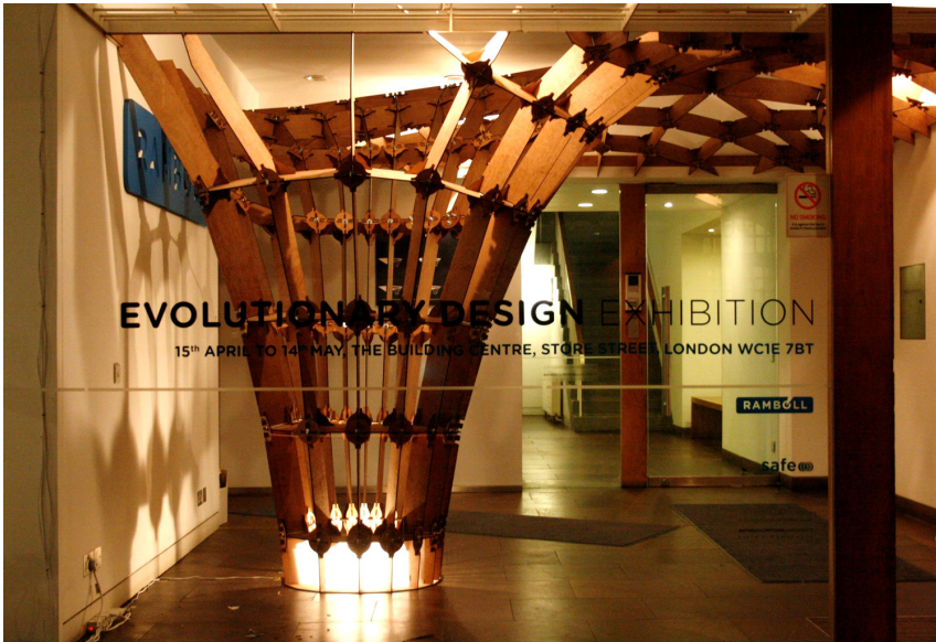
Figure D.4: Final constructed gridshell
