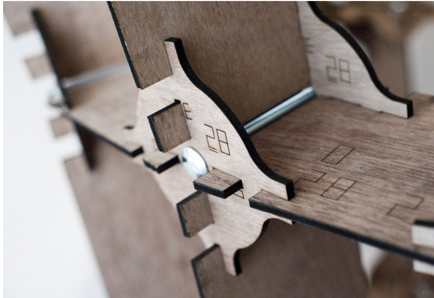
Figure 3.9: Node detail on the London Foyer Sculpture
