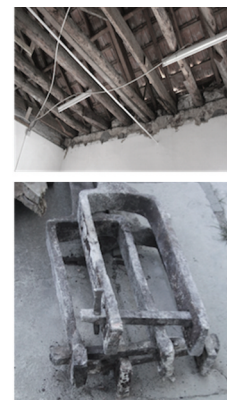
Figure 8. Improvement of the wall-to-roof connections using steel tie rods. Adapted from (Tiago Miguel Ferreira, Maio, and Vicente 2017).
