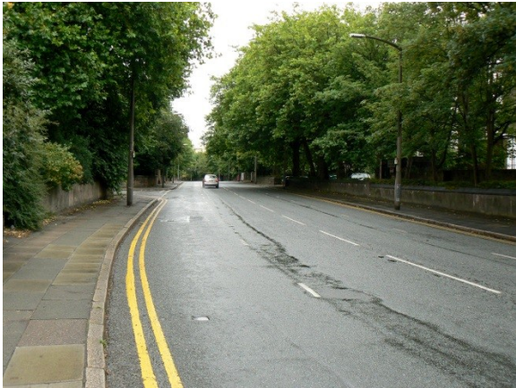
Two lanes, both of which are general traffic lanes, with a centre-line ('dual lane')
