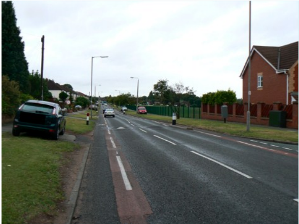
Two lanes, one of which is a cycle lane, with a centre-line ('cycle lane')
