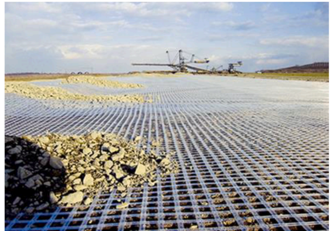
Fig. 9. Soil reinforced with Geogrids(Kiganda, 2016).
