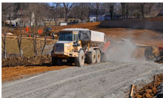
Fig. 13. Cement stabilisation process in road construction (Pleasant Construction, Inc).
