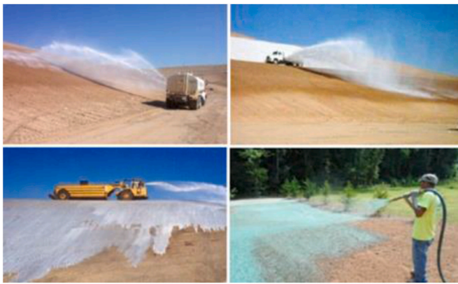
Fig. 18. Application of liquid polymer in road construction (Soil stabilisation Innovations).
