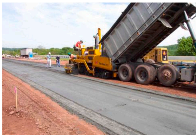
Fig. 15. Fly ash stabilisation process in road construction (Beeghly et al., 2003).
