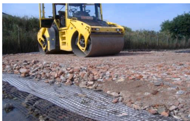
Fig. 16. Construction and demolition waste, Geogrid and textile used in road construction(ABG Geosynthetics).
