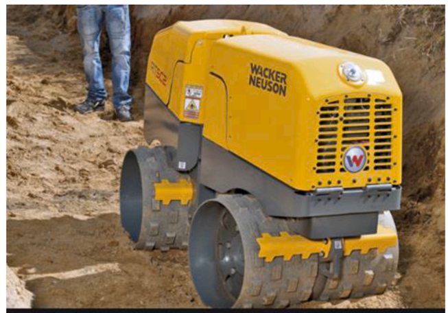
Fig. 10. Compaction process(Compact Equipment).
