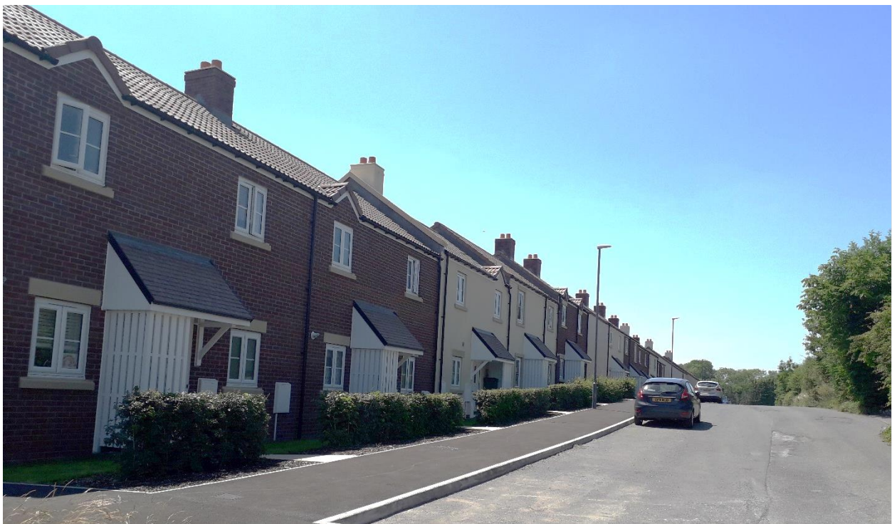
Image MT4: Photograph from site visit (source: authors)
