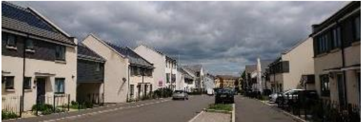
Image CH11: Phase 2 Wood Street (from west end looking east back to phase 1 brick fronted houses in distance). Wide primary street with parking bays, wide kerbed pavements and ‘through’ access to parking at rear. Two and three storey semis and terraces. Mainly rendered finish with some blue/grey brick detailing at first floor, plastic wood effect paneling over the rear access tunnel. Note the stone sill with deeper reveal grey fenestration, parapet gabled ends and railed front gardens.
