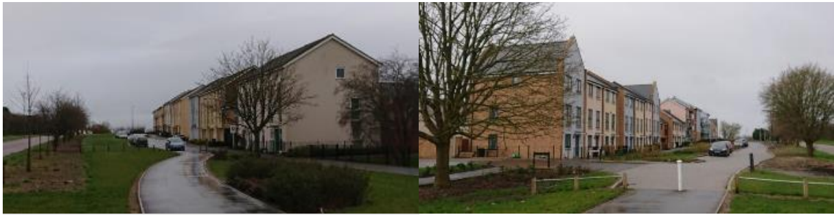
Image CH9: Highwood Road Phase 1 (looking East)
