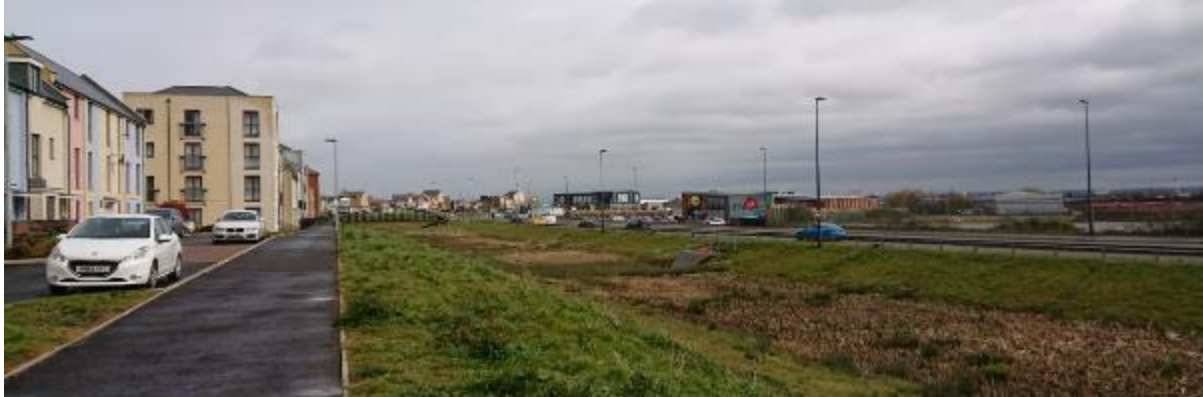
Image CH18: The Hayes Way landscaping scheme with footbridge crossing the swale in the distance
