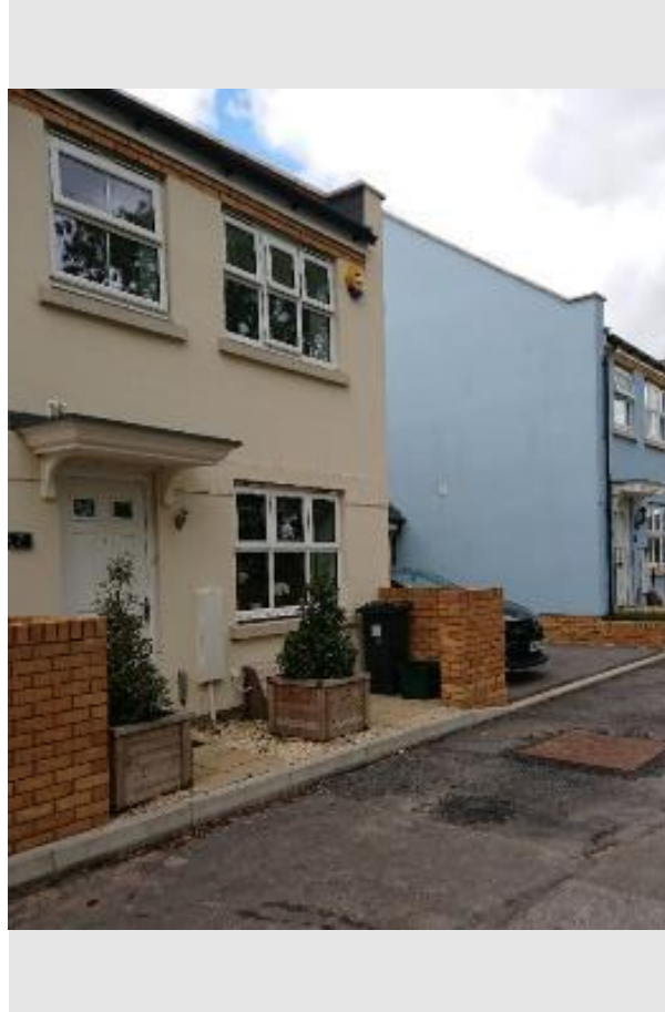
Image CH13: An 'L' shaped brickbin storage area helps to maintain a tidy appearance at the front of dwellings in Phases 2 and 3.
