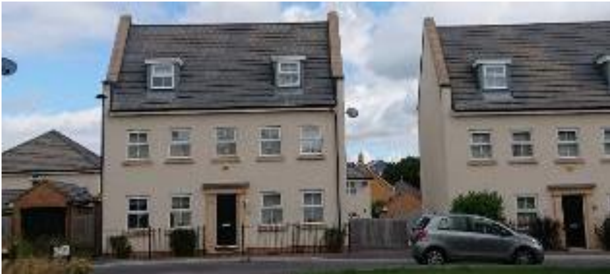
Image CH6: The ‘Georgian style’ of the woodlands phase. A three storey detached town house with flat dormer roof windows, capped parapet gables, symmetrical fenestration (white plastic double-glazing with reconstituted stone lintels), cream render finish, central front door (traditional design) with pillar-surround and canopy, front garden metal railings with side access to brick-built pitched roof garage.
