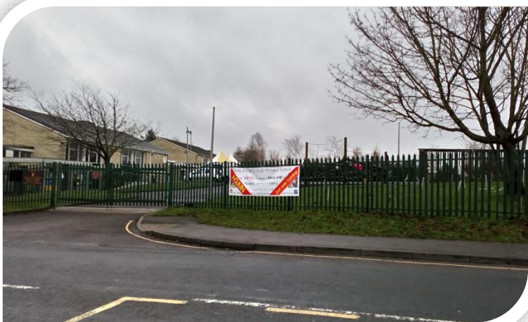
Figure 8 - Nailsworth Primary School
