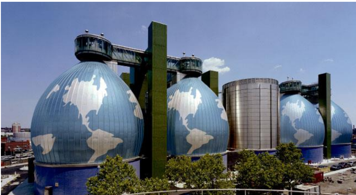
Figure 6. Structural Steel QSDs at Newtown Creek Wastewater Treatment Plant, Brooklyn, New York, USA. (Photograph courtesy Newton Creek WWTP).
