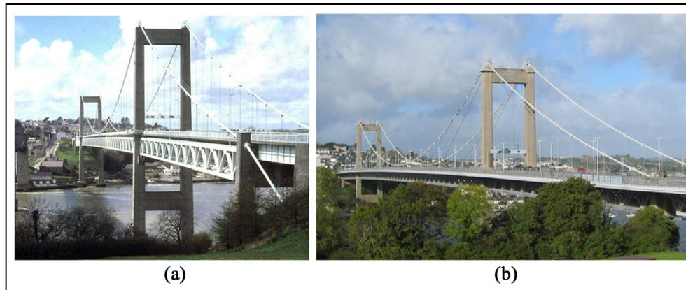
**Figure 2.** Tamar suspension bridge (a) before (1978)<sup>36</sup> and (b) after (2018) its reconstruction in the late 1990s. Note the larger deck and stay cables added in 2001.
