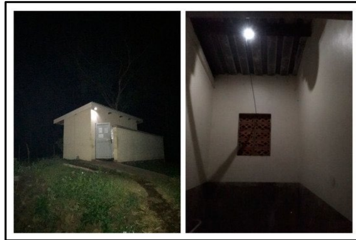
a. PEEPOWER lighting a boarding school toilet at night in Kisoro.
