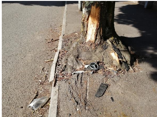
Beddoe Street, damage to tree and debris from apparent car crash.
