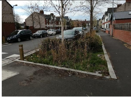
Ashley Street, Sustainable Drainage System (SuDS).
