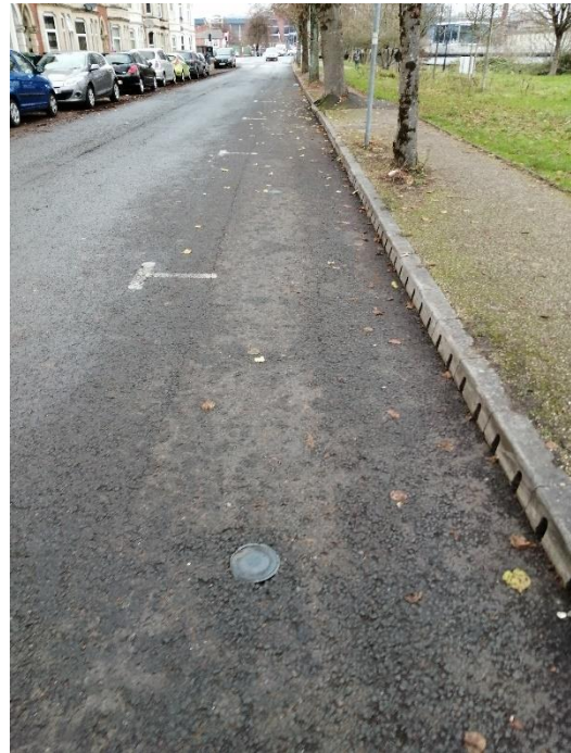
Tomos Street, on street parking and sensors in ground for parking mobile apps.
