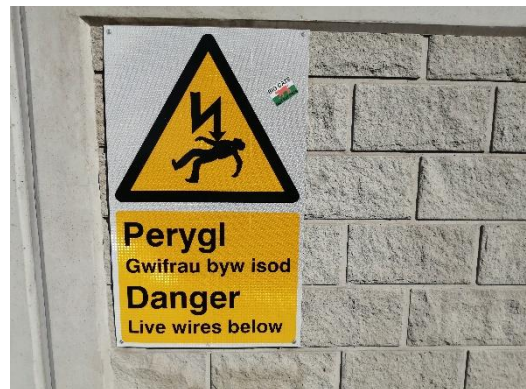
Steer Street, railway electrical warning.
