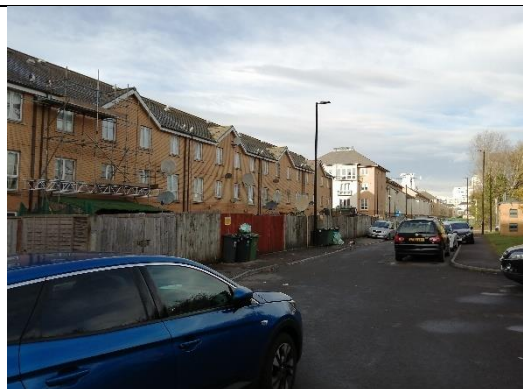
Campbell Street, satellite dishes all on street away from main public street due to legal restriction.
