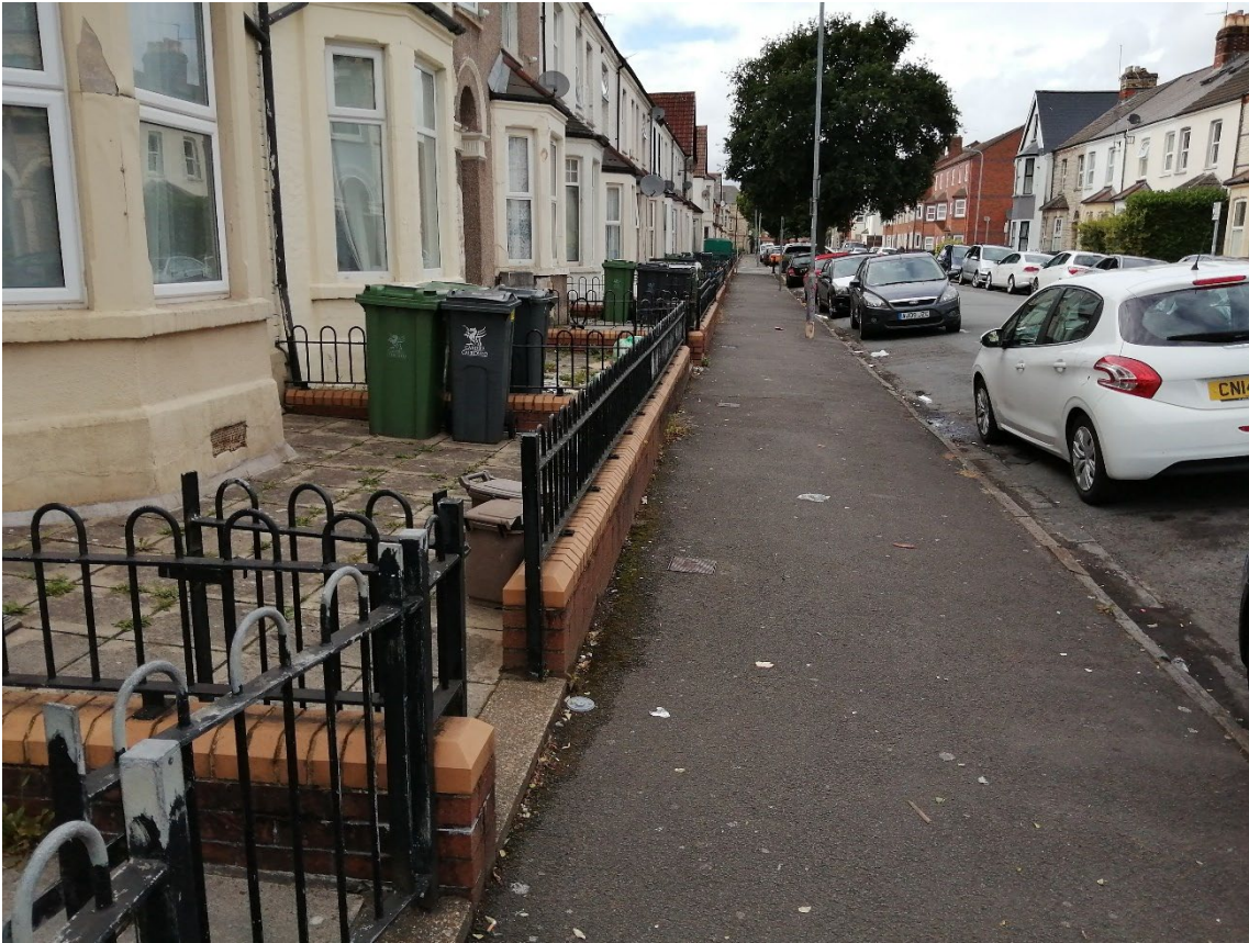
Figure 31: Philippa Street, evidence of previous regeneration intervention to standardise garden walls and railings
