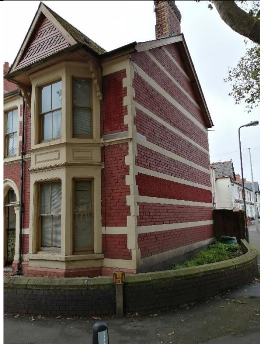
Cadwaladr Street, patterned brickwork.
