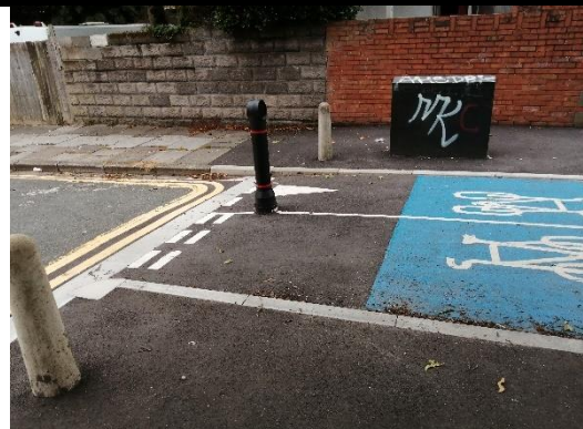
Philippa Street, existing dead end but now with dropped kerbs and route through for cyclists and pedestrians.
