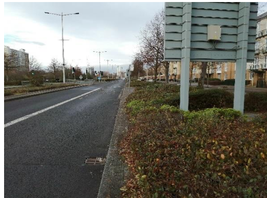
Tomos Street, much larger lighting of a highway type not a street type.
