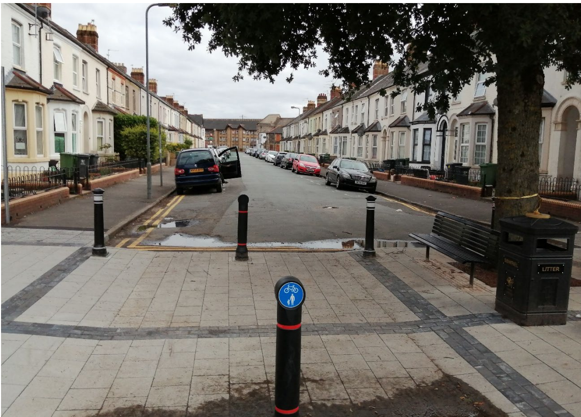
Figure 52: Philippa Street, dead end with recent new modal filter for walking and cycling, new bench, identified as location of fly tipping
