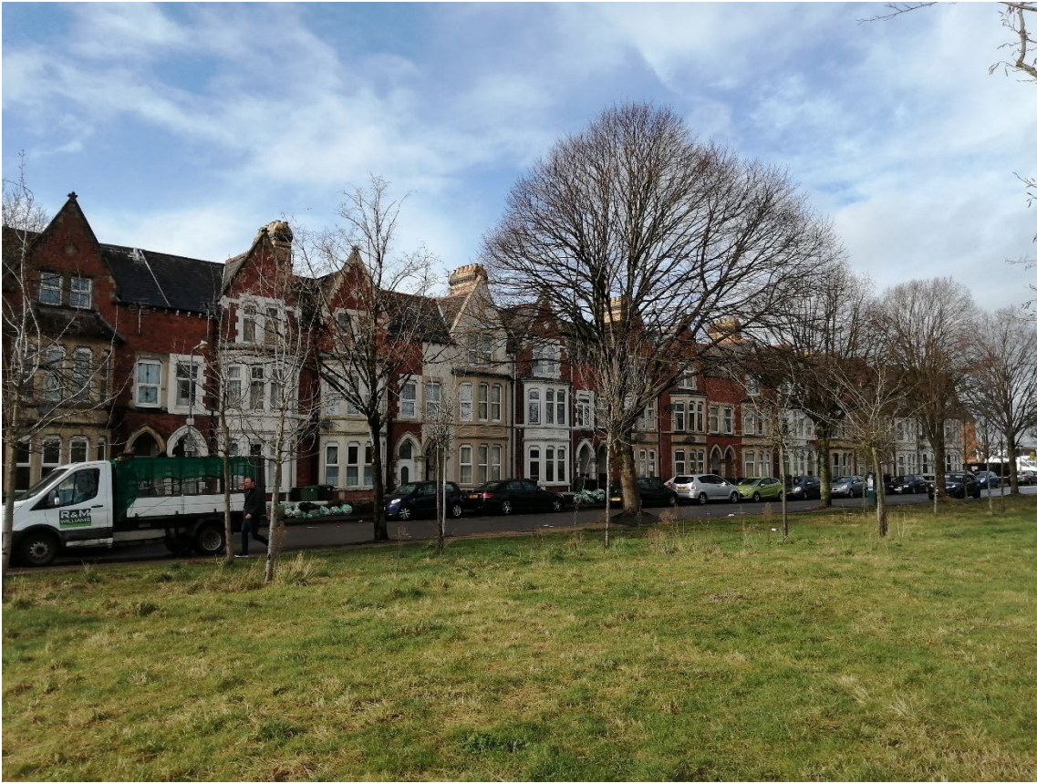
Figure 38: Tomos Street, park forming one side of the street (river behind)
