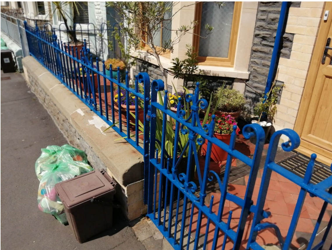
Figure 29: Simpson Street North, example with small front garden / yard
