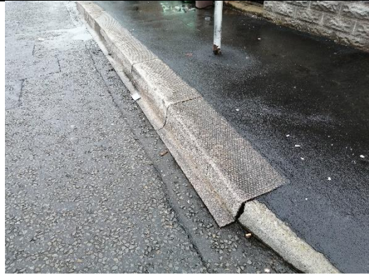
Hester Street, raised kerb associated with bus stop.
