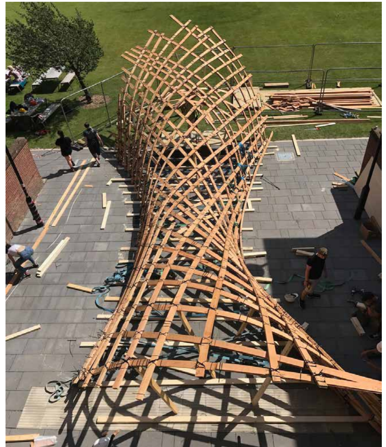
23 (Previous) Completed Watchtower.
