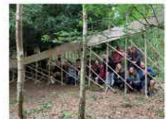
20: Participants, completed structure 21: (Below) Completed Structure
