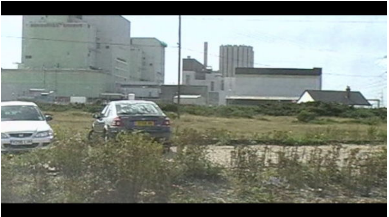
Figure 12: Last frame of Missing Derek showing Dungeness power stations
