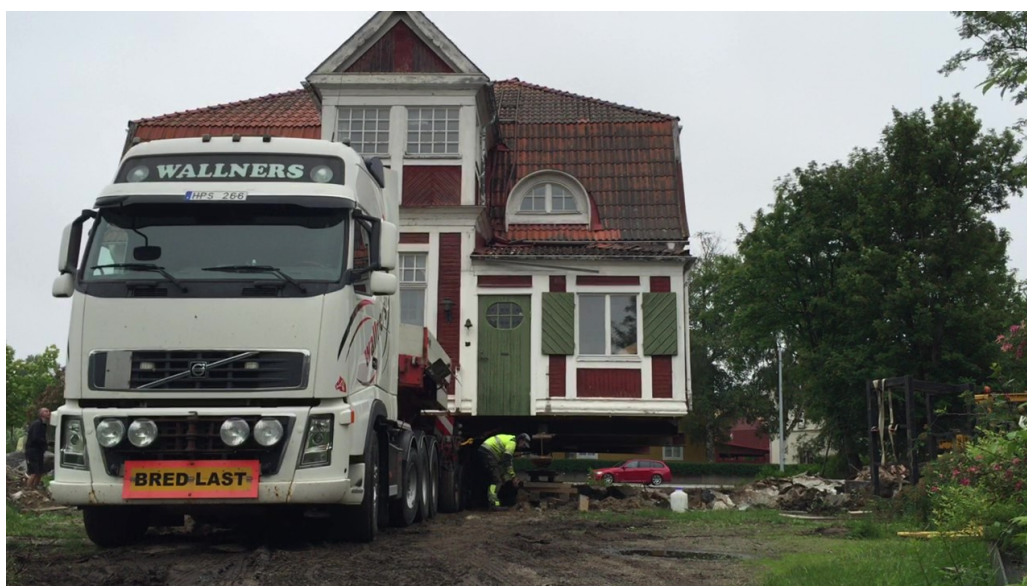
Figure 2. Historic house being lifted, to move from its site at Teg in the city of Umeå Film Still Tonia Carless 2021
