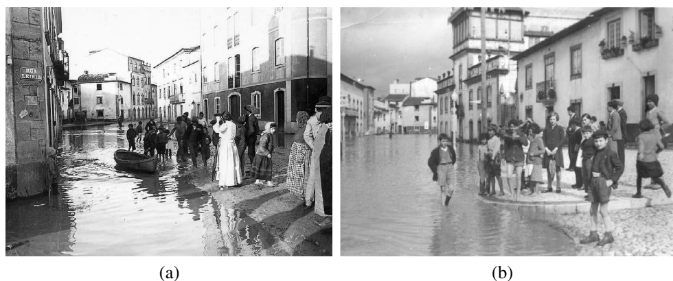
FIGURE 1 Flooding in the city centre: (a) 1915–1931 Rua Everard; (b) 1950–1957, Praceta Alves Redol. Source: (Memória Digital de Tomar, 2013).
