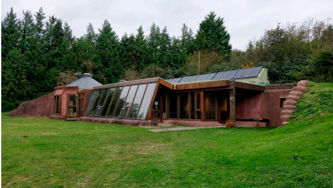
Figure 1: Exterior of Earthship Brighton with slanting glass walls flanked by Earth-rammed tyre walls and solar panels on the roof (Booth et al., 2021) (Credited to Sona Rasheed)
