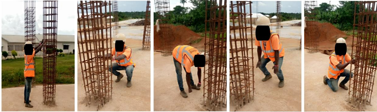
465 466 Fig. 3. Field experiments of different types of awkward working postures: (a) Overhead working; 467 (b) Squatting; (c) Stooping; (d) Semi-squatting; and (e) One-legged kneeling
