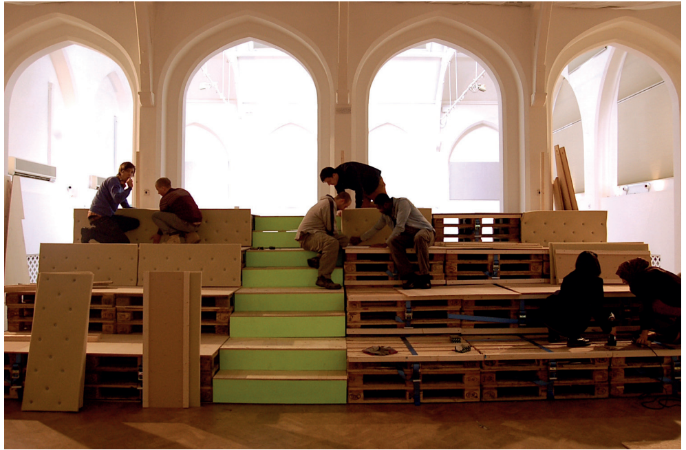
Figure 3: The Flatpack Palais under construction (Alessandro Columbano 2013).
