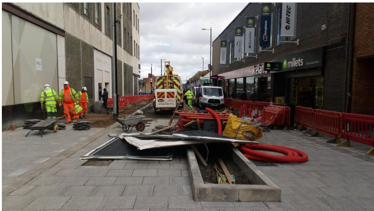
Figure 3: Groundworks at York Road Site
