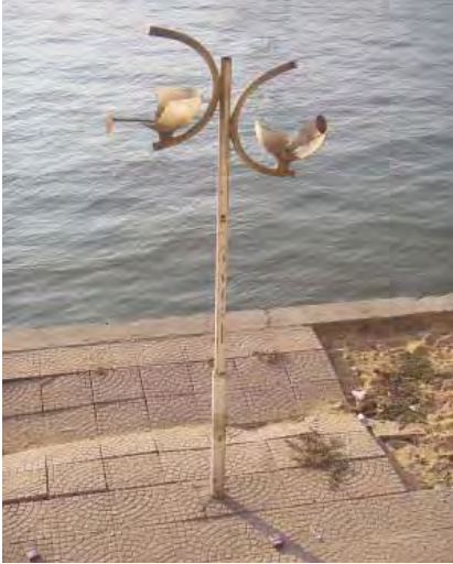
FIGURE 149. Broken lampposts and crumbling pavement along Roda Island's formerly grand sidewalks
