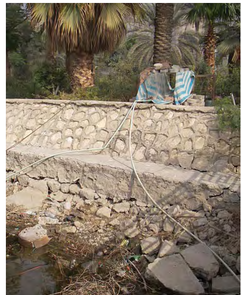
FIGURE 113. Unused vegetated terraces in Maadi
