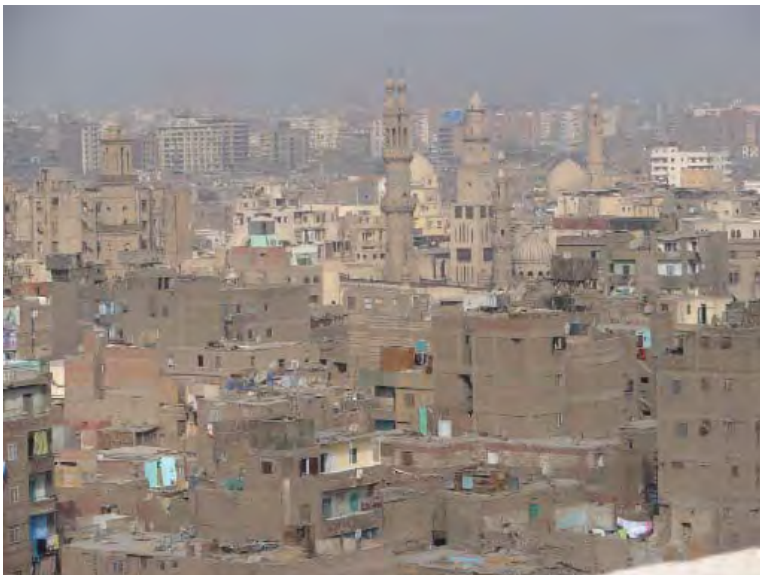
FIGURE 8. Al-Darb Al-Ahmar District
