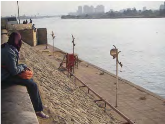
FIGURE 62. Steep concrete walls serve as riverbanks on Roda Island
