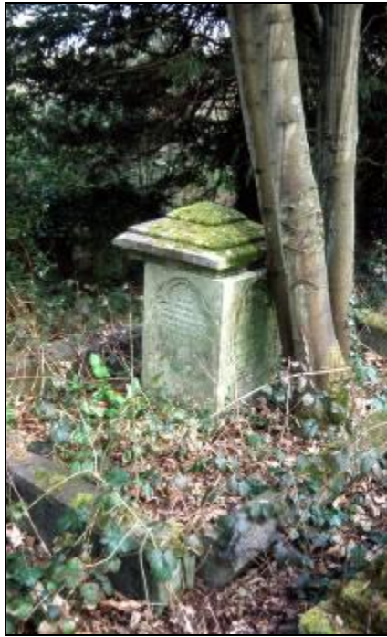
Figure 10. wild tree seeded in a grave bed and slowly displacing masonry.
