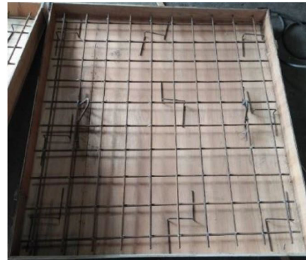
(b) Lower slab reinforcement
