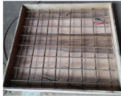
(a) Upper slab reinforcement
