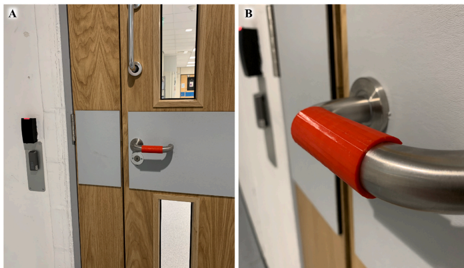
Fig. 15. The original sample of 3D printed door handle socket from a (A) distant and (B) close-up view.
