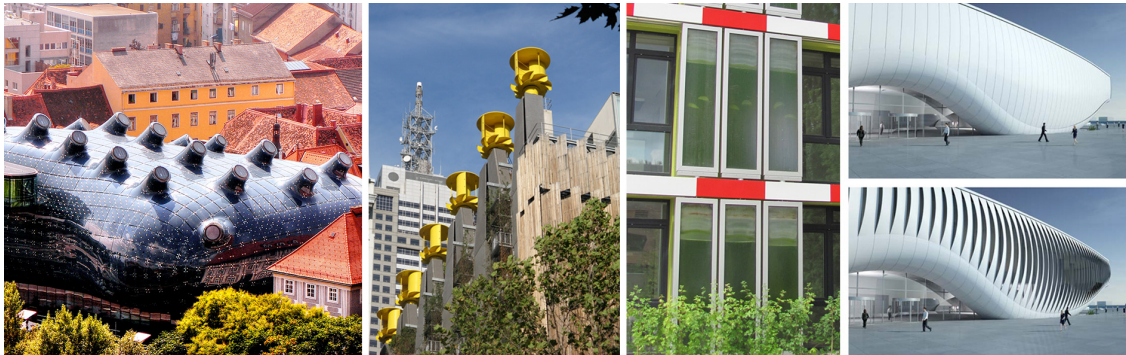
Figure 1. From left to right: the free form envelope of the Kunsthaus in Graz, used with permission ©Heribert Pohl; the turbines of Council House 2 in Melbourne, courtesy of Nick Carson; the façade of the BIQ building consisting of algae filled panels, used with permission ©NordNordWest; the bending façade of One Ocean Thematic Pavilion, photos courtesy of SOMA.
