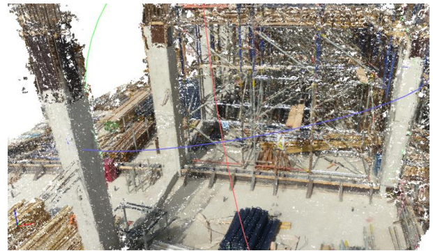
Fig. 2a. Point cloud built from captured photos for columns
