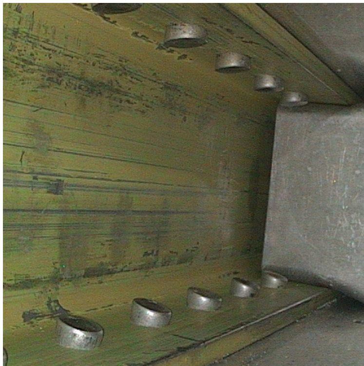
Figure 4.3: A wing spar of the test aircraft (photographed during inspection in February 2014)
