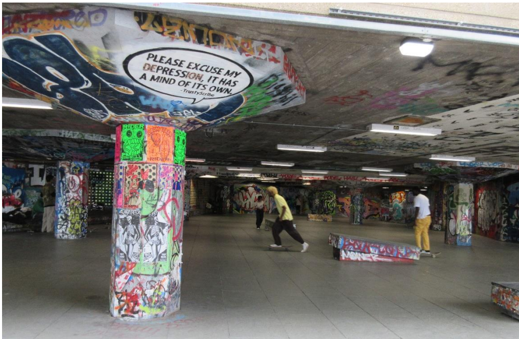
Fig3 South Bank centre undercroft colonised by skateboarders adapted to their own concept of beauty
