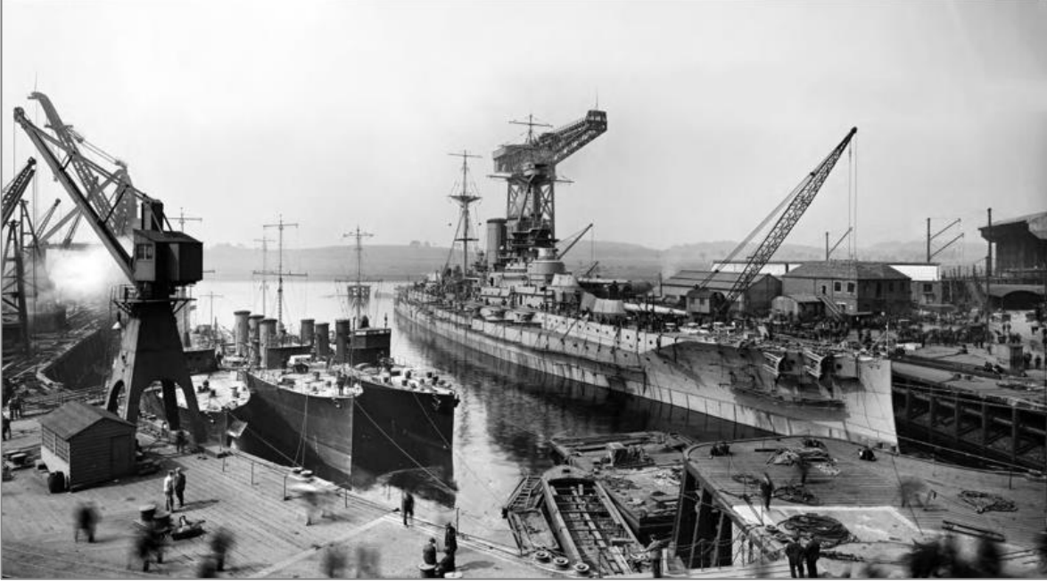
"HMS Barham and the destroyers Mons and Medusa, being fitted out at Clydebank, July" https://www.pinterest.com.au/pin/485544403568438101/
