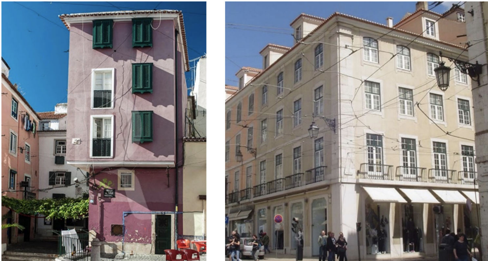
Figure 5. Unreinforced masonry buildings in the Lisbon Metropolitan Area: ‘Pre-Pombalino’ buildings (a) and ‘Pombalino’ buildings (b).
