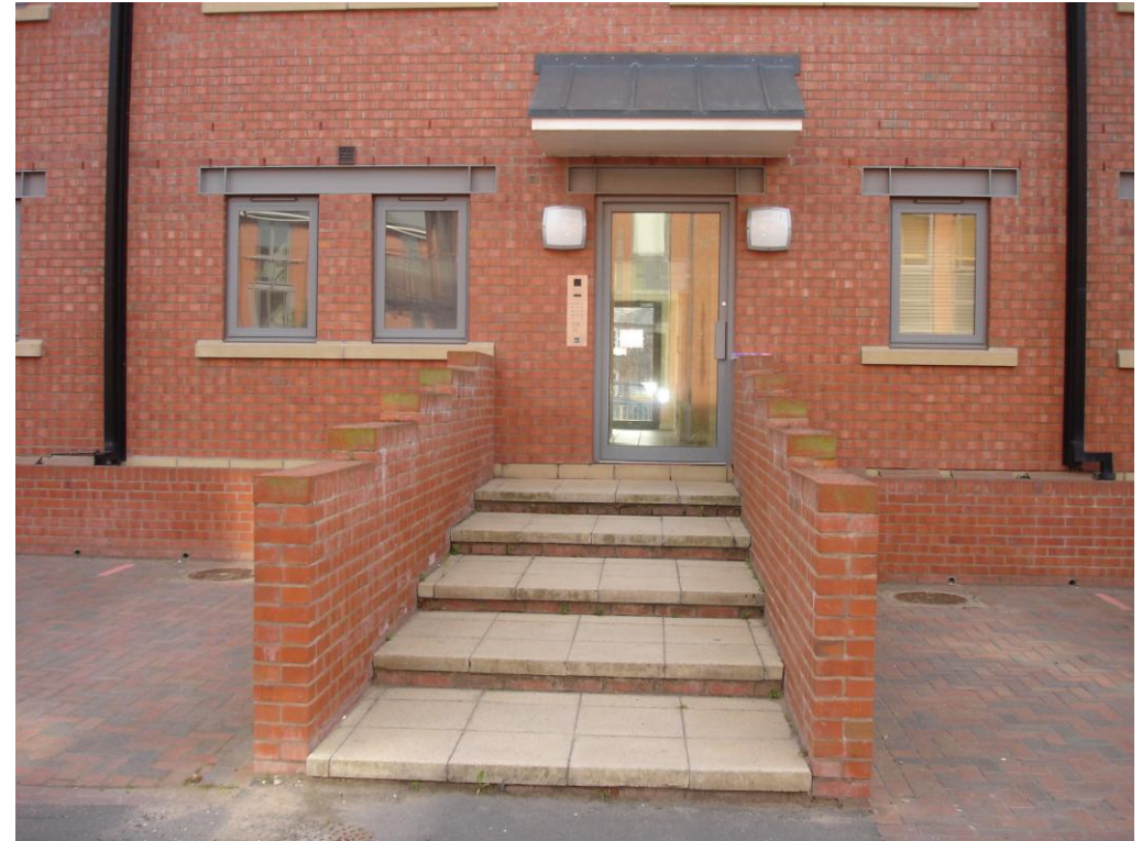
Figure 8: New residential building under construction in 2005
