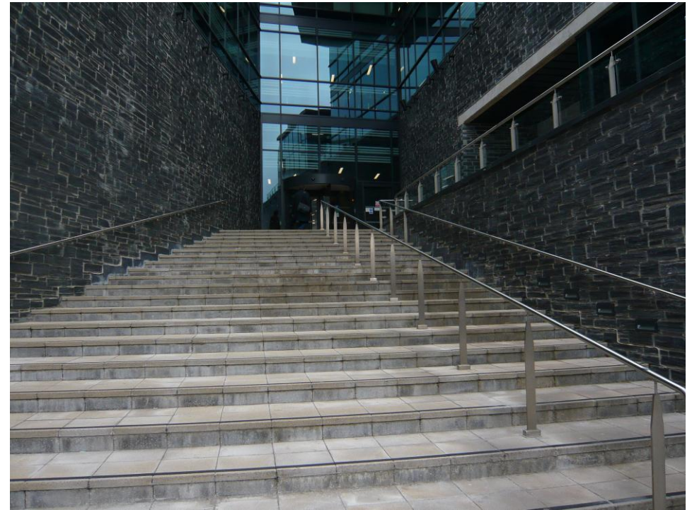
Figure 21: segregated stepped entrance to Plymouth School of Architecture (The route for wheelchair access is elsewhere. Steps are often used to “add drama” to the entrance experience).
