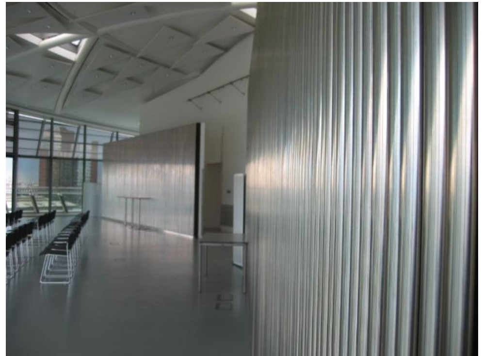
Figure 19: Inadequate colour contrast and confusing reflective surfaces in conference hall to modern public building
