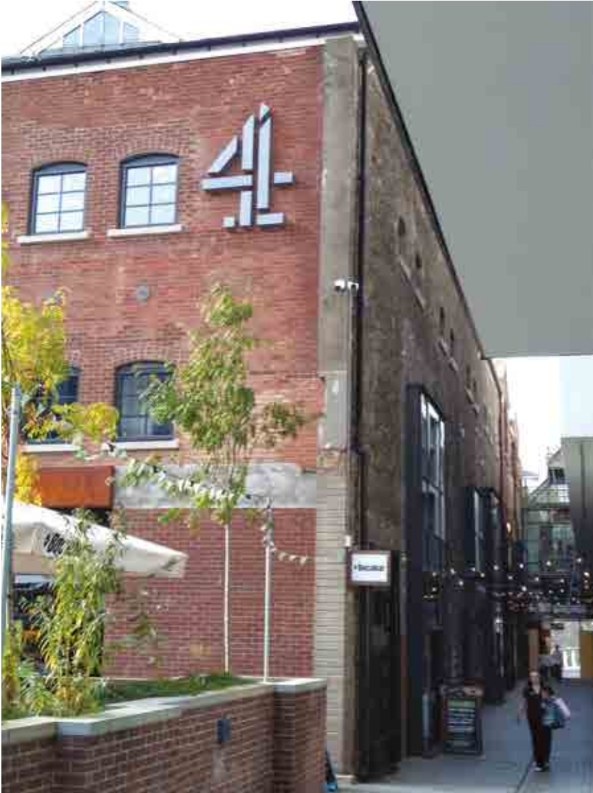
Figure 13 Exterior of Channel 4's offices in Finzels Reach; Photo: Steve Presence
