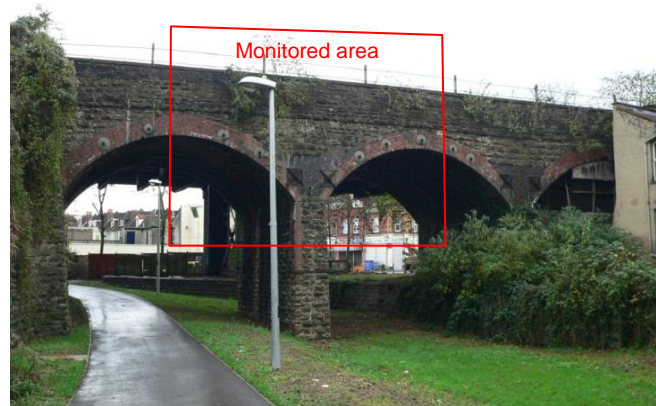
Figure 6: Railway bridge with the monitored area
