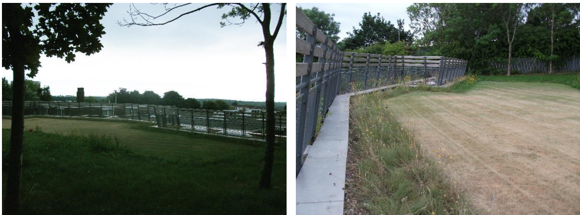
Angram Bank Children's Centre, Sheffield. Courtesy of the Green Roof Centre.
