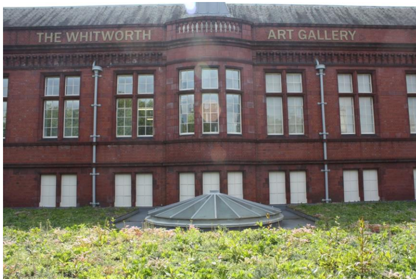
Green roof at the Whitworth, University of Manchester. Photo courtesy of City of Trees.
