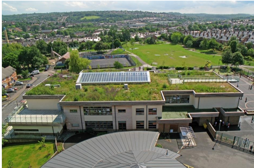
Sharrow School, Sheffield, Courtesy of the Green Roof Centre.
