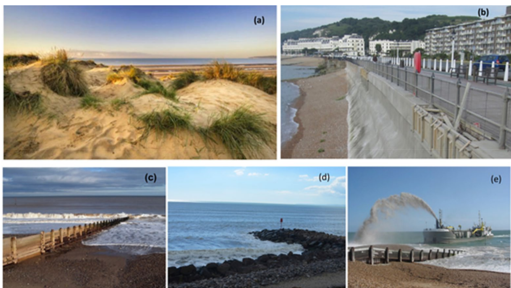
Figure 2. (a) Sand dunes; (b) Sea wall; (c) Groins; (d) Revetments rock armor, (e) Nourishment. Source: Bramley & Teal (2020); Mackley (2014); Wright (2008); Eastern Solent (2015).
