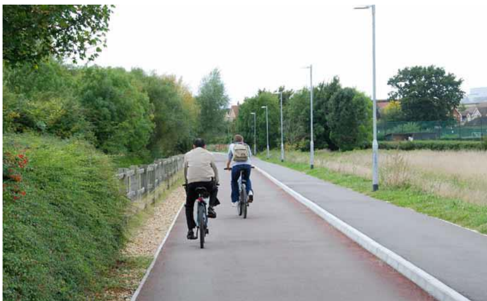
Image 2 - Shared path segregation by kerb
