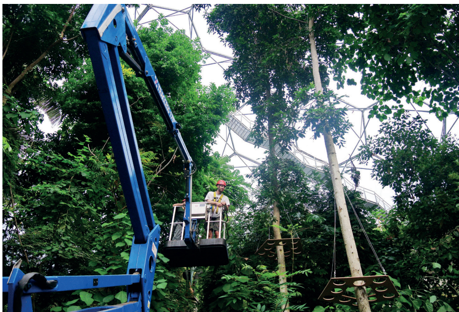
Fig. 5 Installing the fernarium using a cherry picker. The platforms are suspended around two Hopea odorata trees using galvanised steel wire attached to the roof. Photo: J. Donald.
