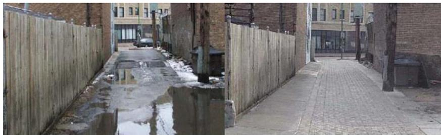
**BEFORE:** Alley with impermeable pavement and poor drainage
