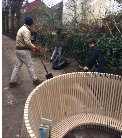
Figure 7. Community site clearance day, Ebenezer Gate, Bedminster, Bristol (Image: Hands-on-bristol, 2016).
