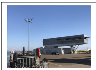
Fig.6 Weather Vane erected on site
