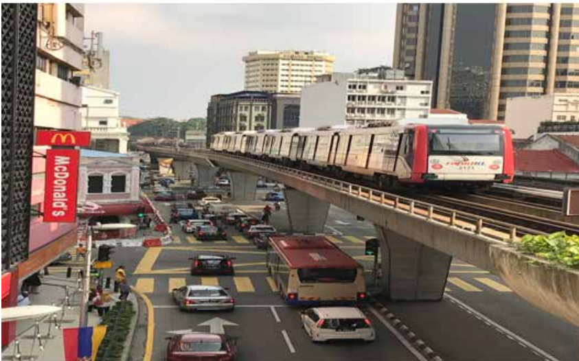
Figure 17: LRT on Track in Kuala Lumpur City Centre.
