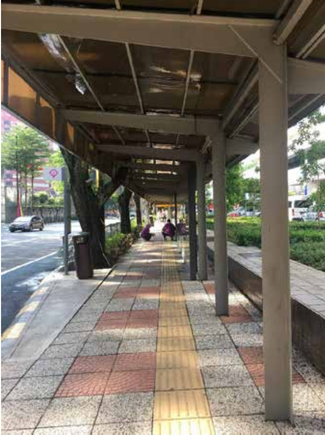
Figure 19: Tactile Pedestrian Walkway – Jalan Bukit Bintang, Kuala Lumpur.
