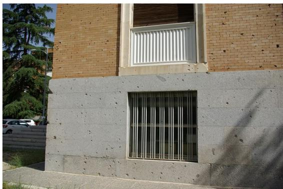
**Fig. 13** Overall view of an area of the building showing ballistic impacts
