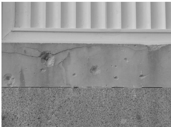
**Fig. 14** Impacts of different sizes in a window ledge. Smaller ones, which are likely the result of small size shrapnel, show inside granular disaggregation, while larger ones, coming likely from either rifles or large steel shrapnel, flaking, scaling and loss of fragments
