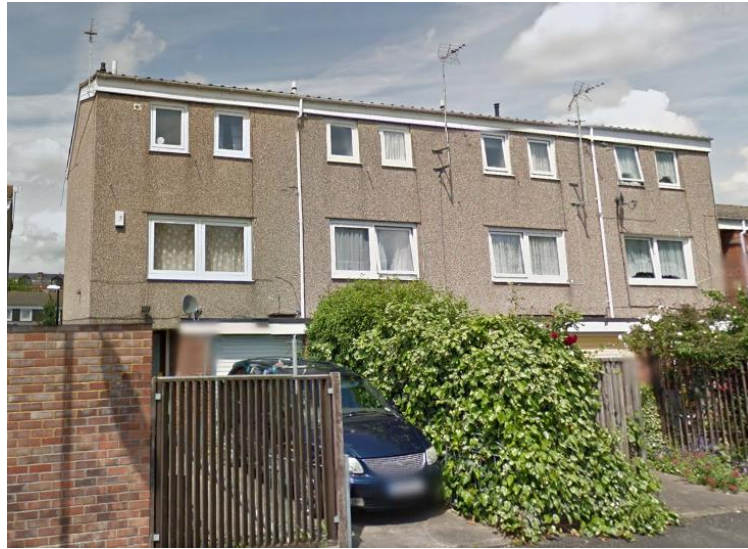
Figure 1: building with house 1
