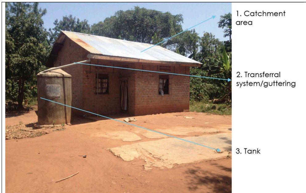
Figure 2. Schematic indicating basic configuration of domestic rainwater harvesting systems in Uganda. Source: the authors.
